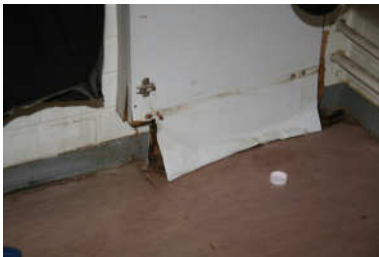
Before upgrade of Procedure Room
